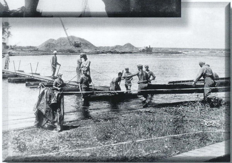
Pontoon bridge building on Lake Gatun.
